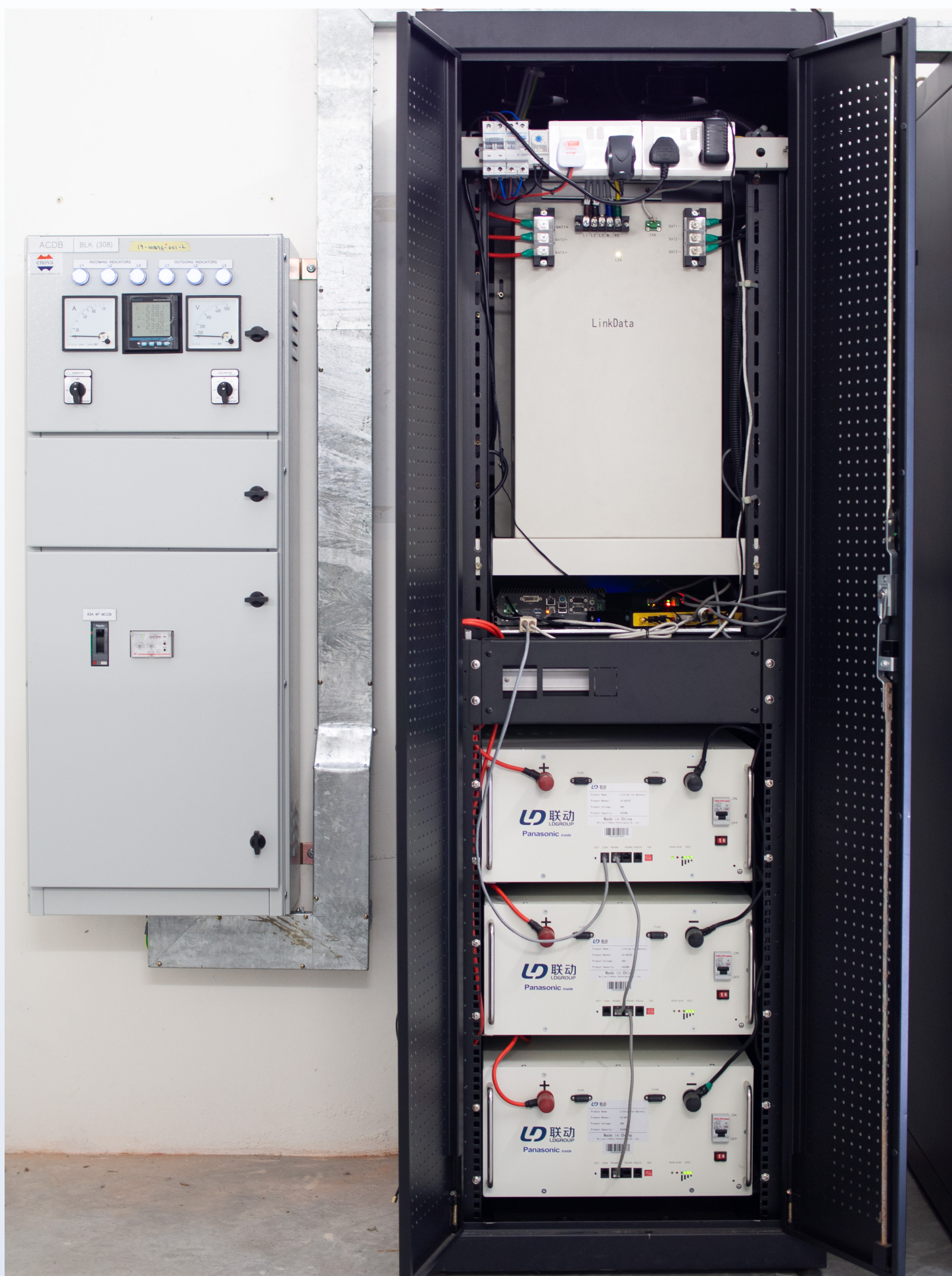
Distributed ESS deployed within a switchroom in Punggol [Photo Credits: Sunseap Group]
